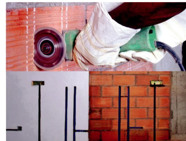
Porotherm Wall with plumbing conduiting before plastering
