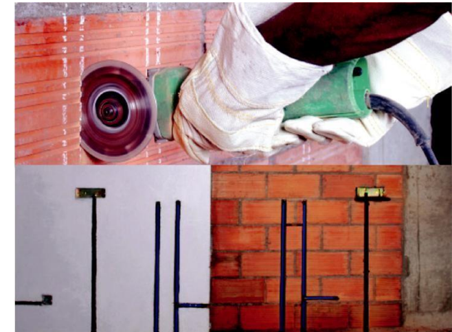
Porotherm Wall with plumbing conduiting before plastering
